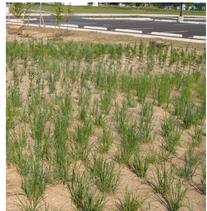
Newly installed Switchgrass ( Panicum virgatum ) in a well-drained bio-retention basin
