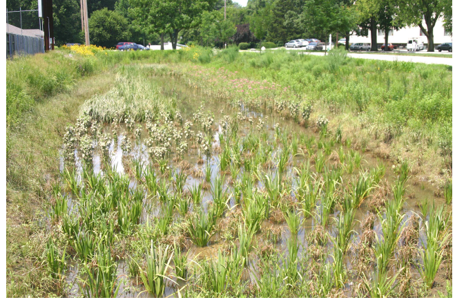
Bio-retention Basins at Butler University recovering from the extreme rainfall of June-July 2008.
