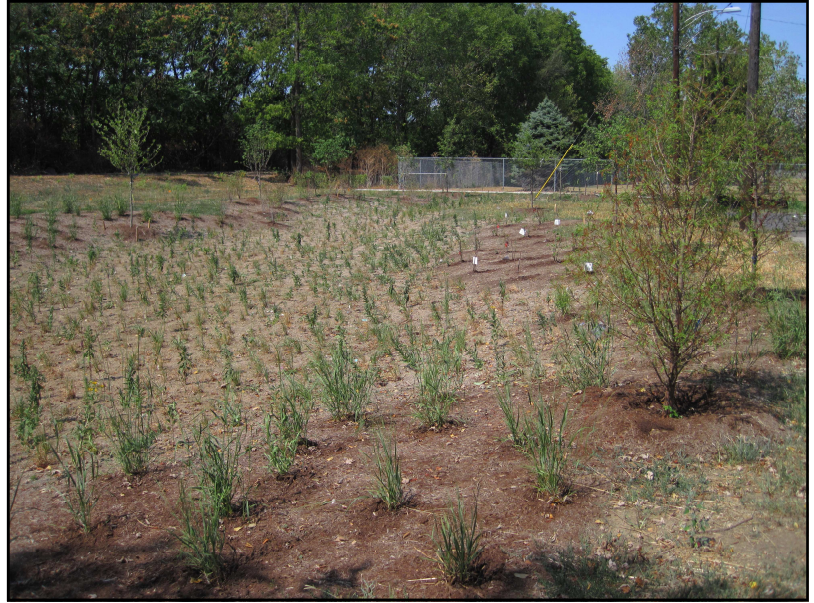
Watering was vital to plant establishment in the Speedway basins during the summer drought of 2012.
